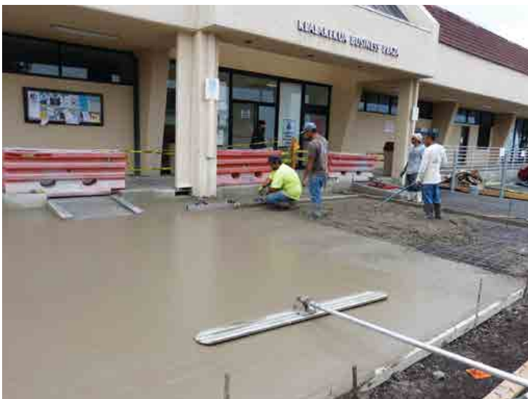
First-pass consolidation (i.e. float) of surface after screeding but before checking the surface with a digital level mag screed.
