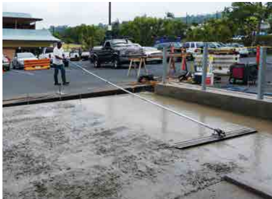
First-pass consolidation (i.e. float) of surface after screeding but before checking the surface with a digital level mag screed.
