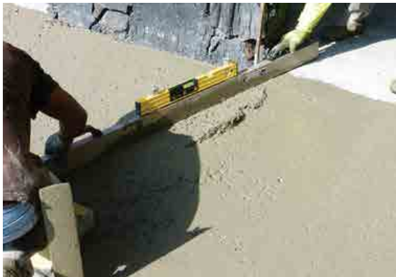
Initial screeding: second-phase bump-cutting using a digital level mounted on a mag beam screed.
