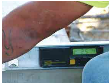
Initial screeding: third-phase bump-cutting dredging method to get cross-slope lower than 2.5 percent.
